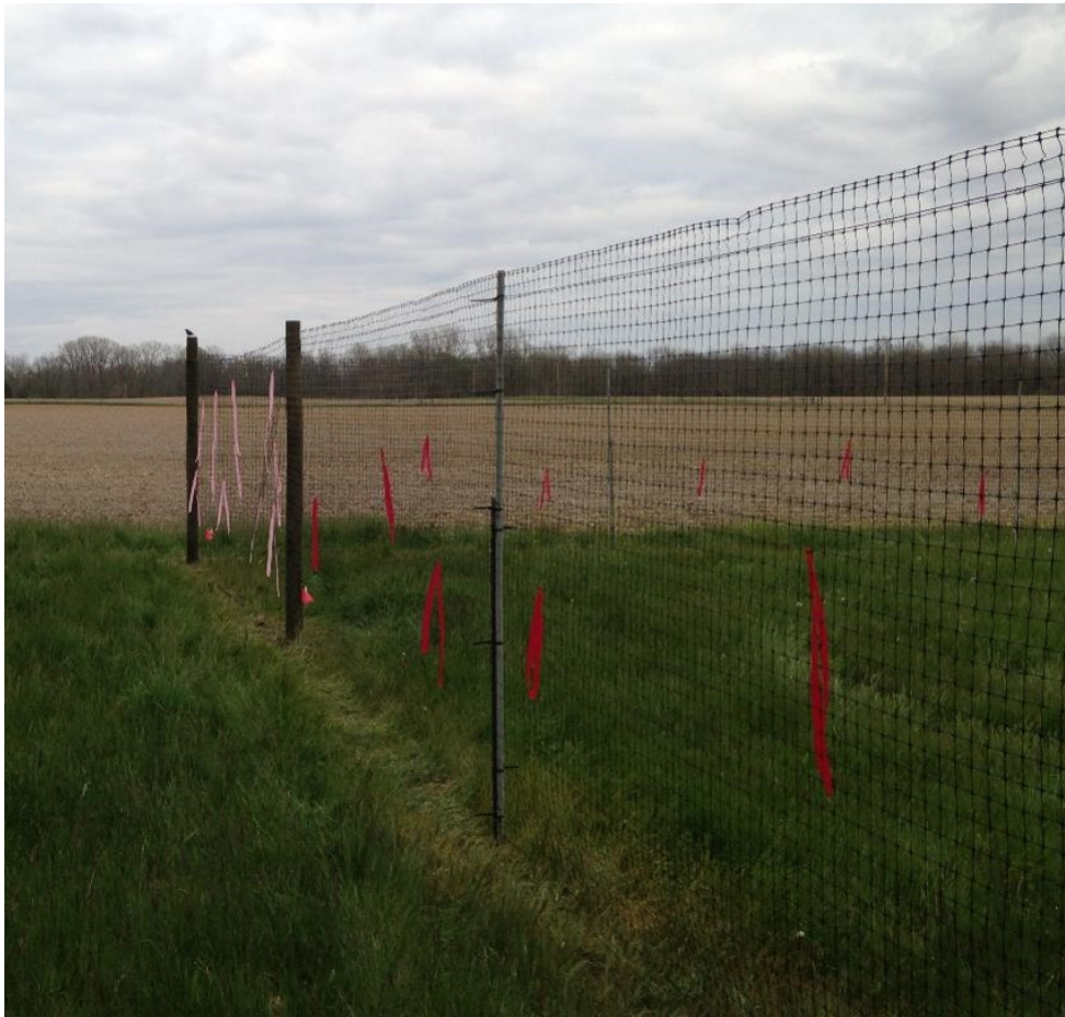
Plastic mesh deer exclusion fence with a combination of wood and metal posts with PVC pipe extensions.
